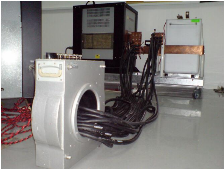
Figure 4. BIM transformer: I 523
