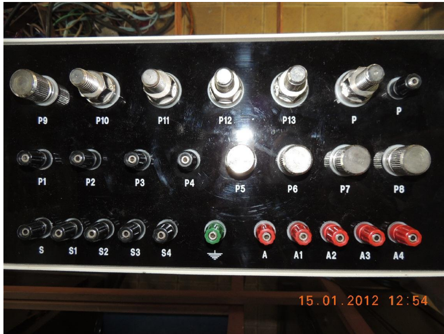
Fig. 3. Up view of the transformer.
