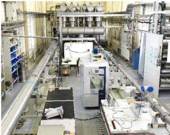
Upstream view to calibration lines
