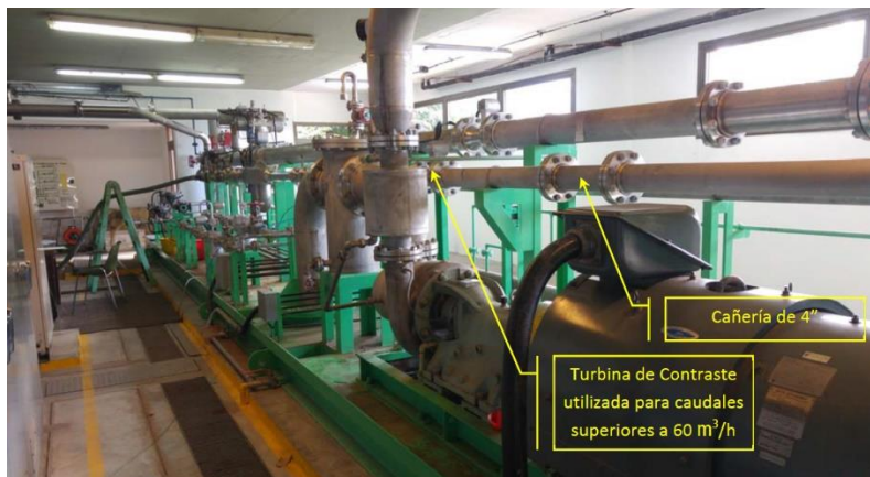
Calibration test rig
