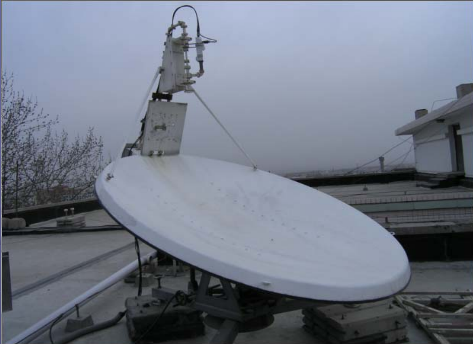
Fig.1 1.8 meters ellipse antenna
