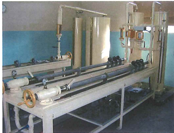
Fig. 7 Installation of the meters
