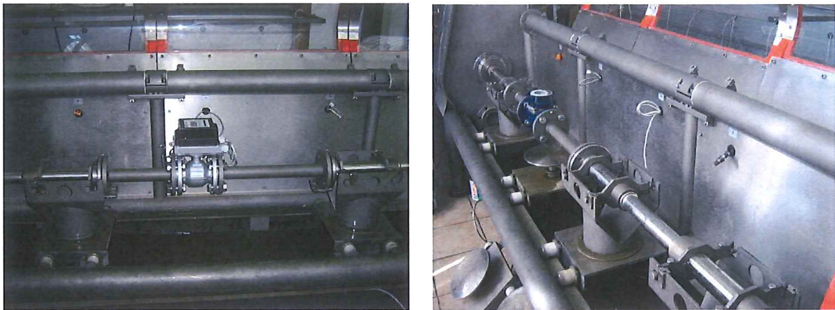
Fig. 9 Installation of the meters
