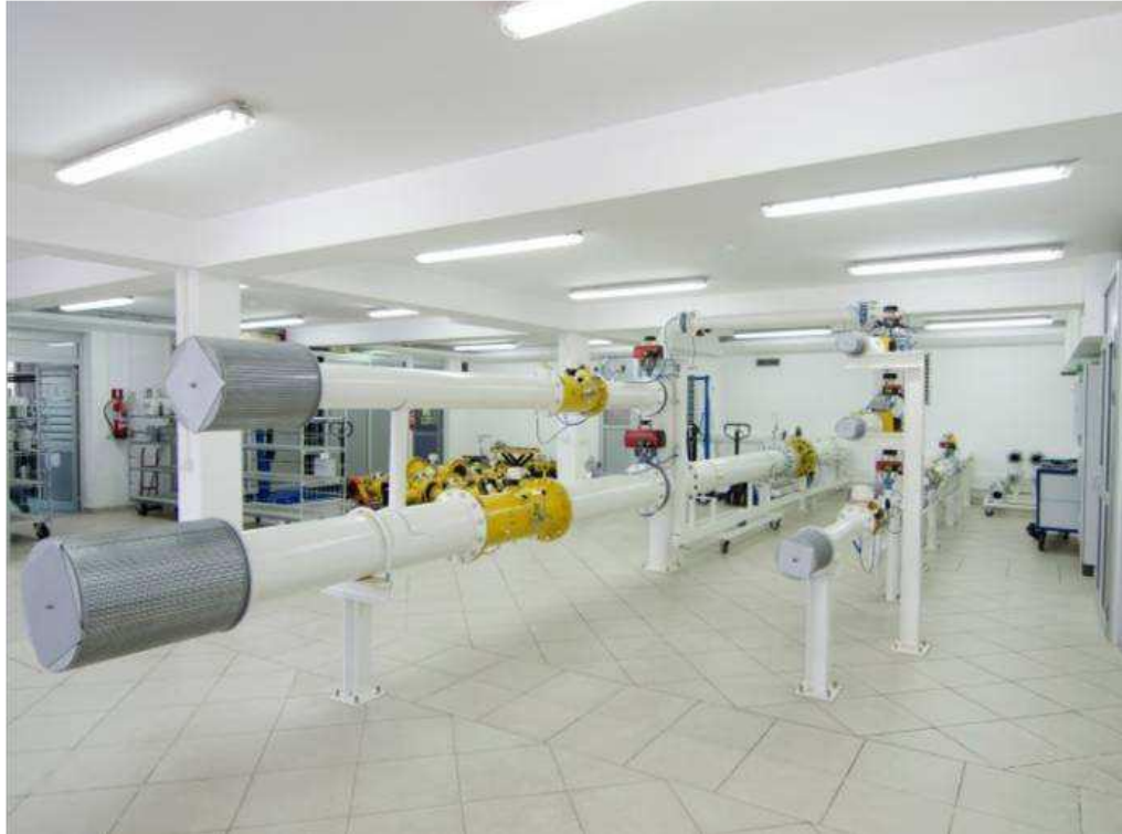
Figure 17 – The general view of LABSAGAS standard facility
