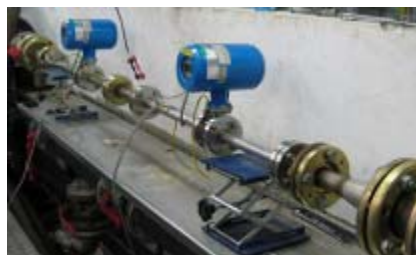
Fig.5.10 Installation of the meters in the CETIAT's test rig (France)
