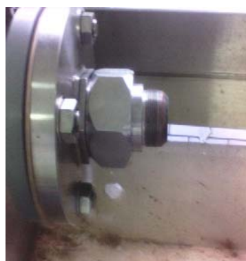
Fig 11. Flange without Reducer Pipe as Protector
