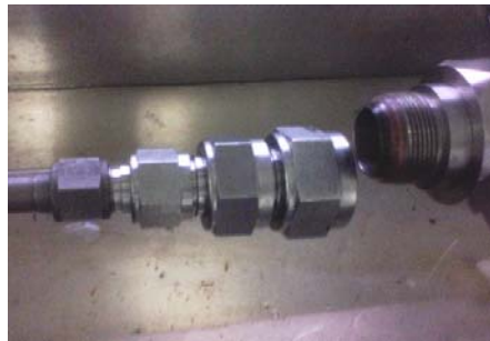
Fig 14. Installation of FT-12 Pipe to the Flange with Mechanical Seal Attach to The Flange
