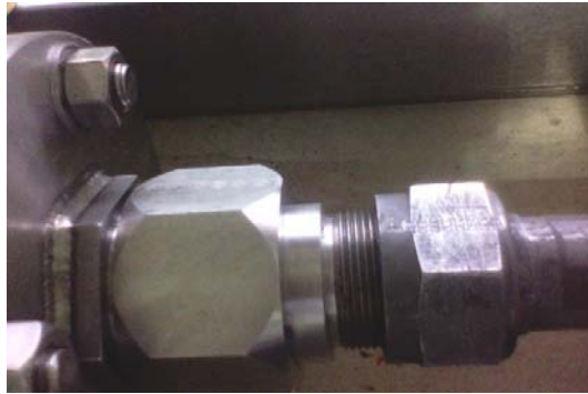
Fig 13. Installation of FT-24 Pipe to the Flange with Mechanical Seal Attach to The Flange
