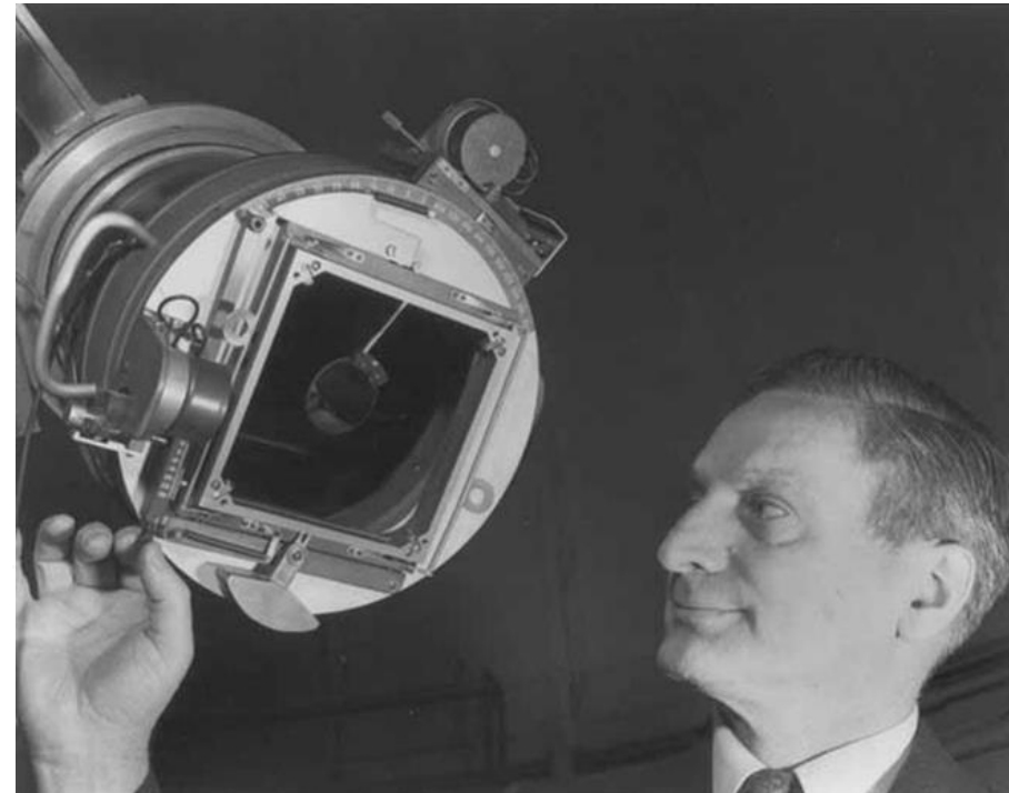
W. Markowitz with dual-rate moon camera for the measurement of occultations of stars by the moon. Photo: USNO
