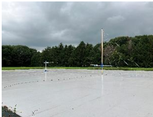
Fig. 10-1 Refreshed open-area test site at NMIJ/AIST.
