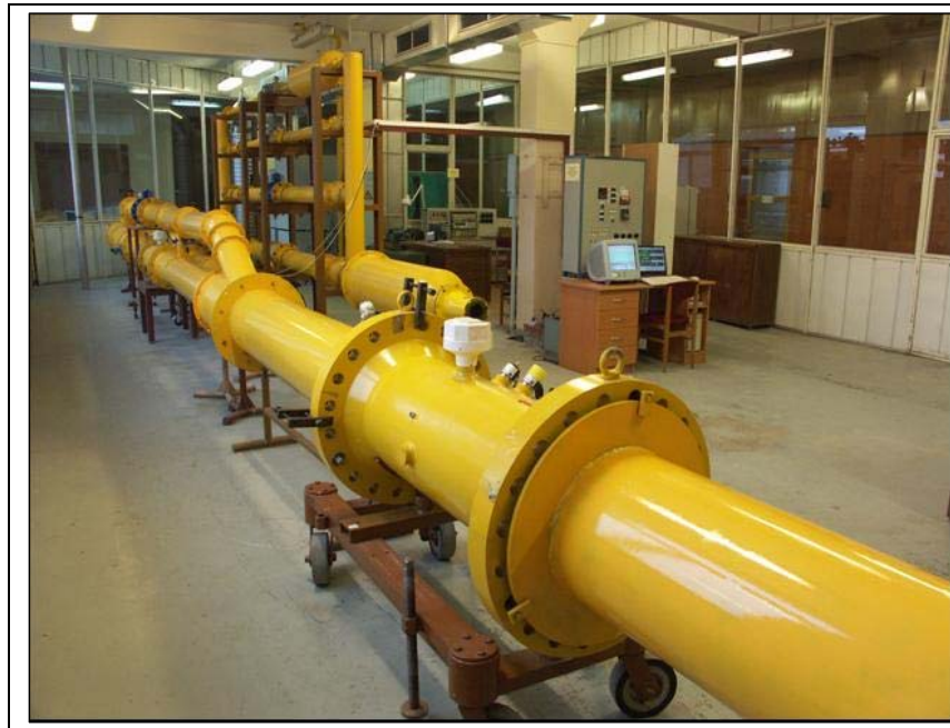
Figure 8 . The general view of the standard facility
