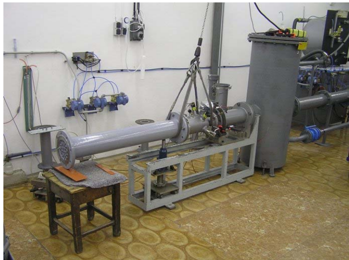
Figure 6 The installation of gasmeter on the test bench
